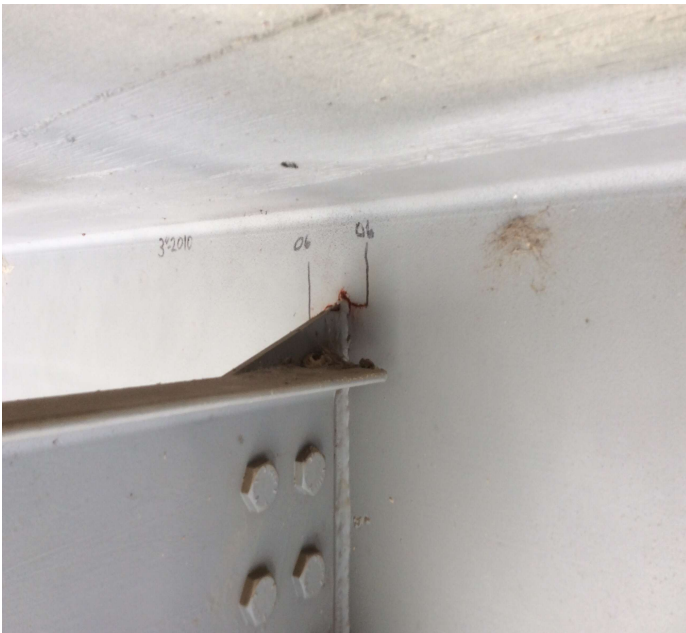
PHOTO 1 Description Typ Cracking in Beams.
