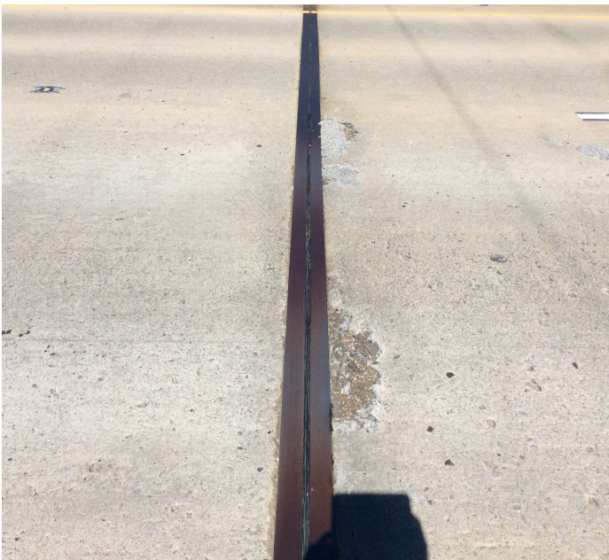
PHOTO 4 Description Typ. Spalling at Joints.
