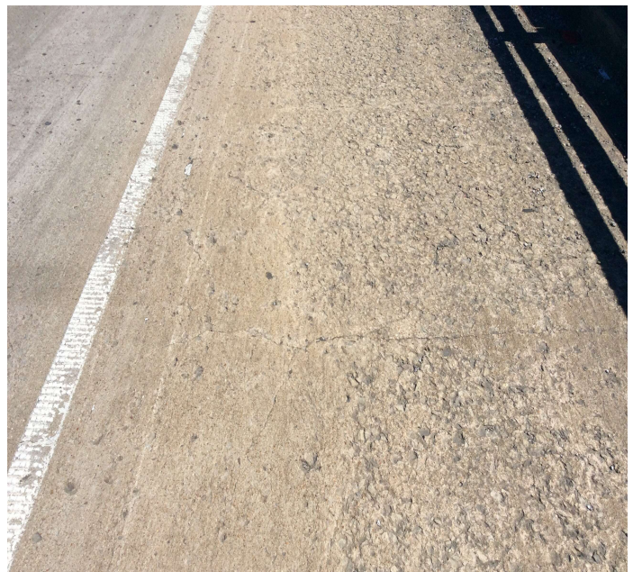
PHOTO 2 Description Typ. Cracking & Scaling in Deck.
