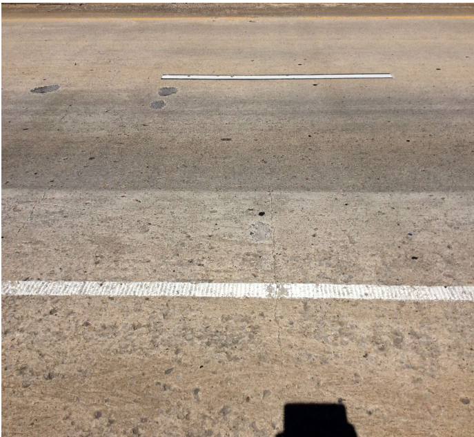
PHOTO 3 Description Typ. Cracking in Deck.
