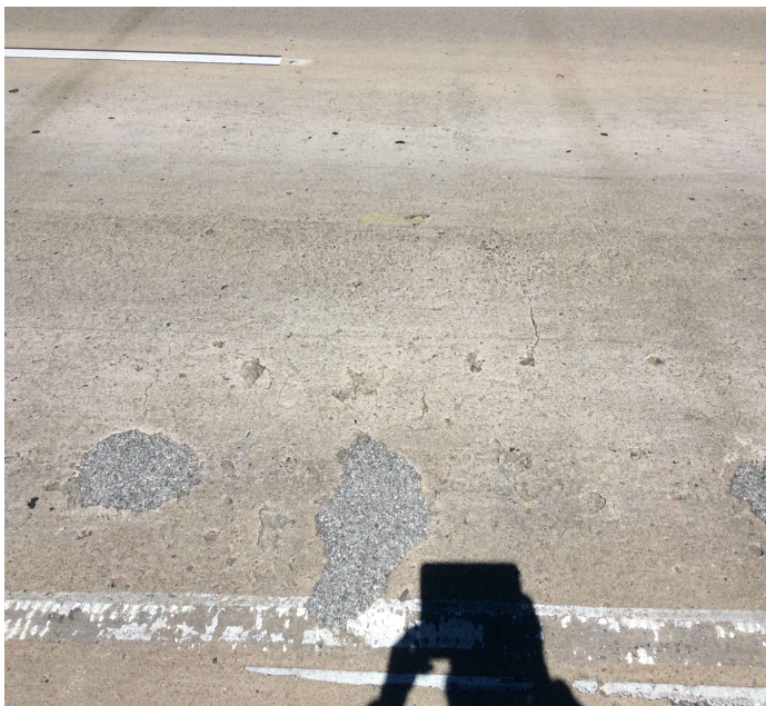
PHOTO 1 Description Typ. Cracking & Spalling in Deck.
