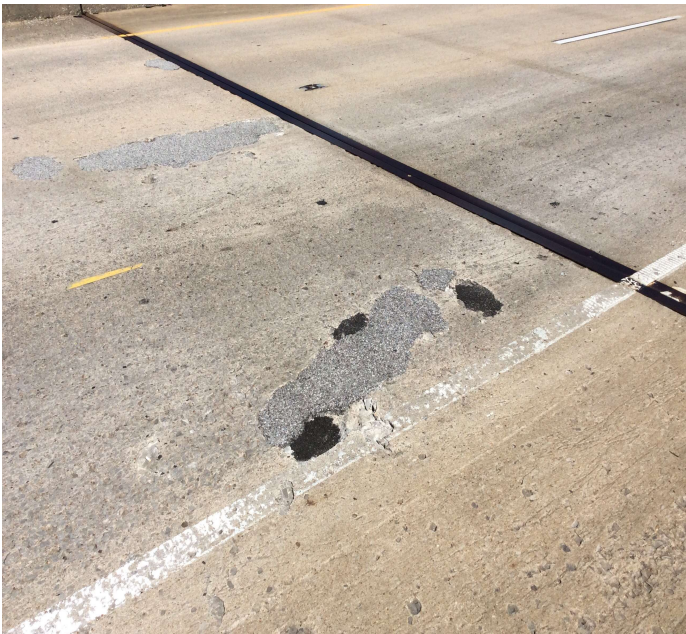
PHOTO 1 Description Typ. Spalling in Span 3.
