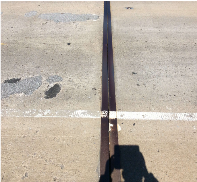
PHOTO 1 Description Seal Failed at Joints.
